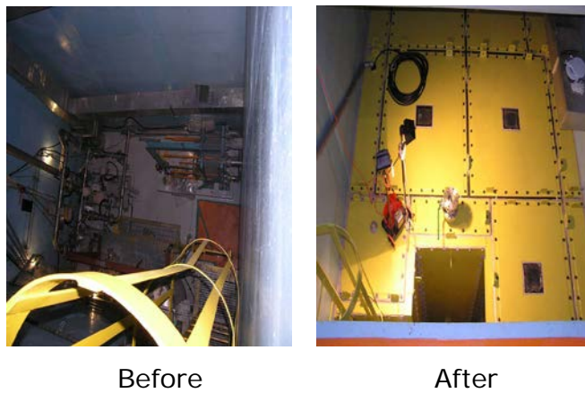
Fig. 2. Top views before and after installation of air tight room
