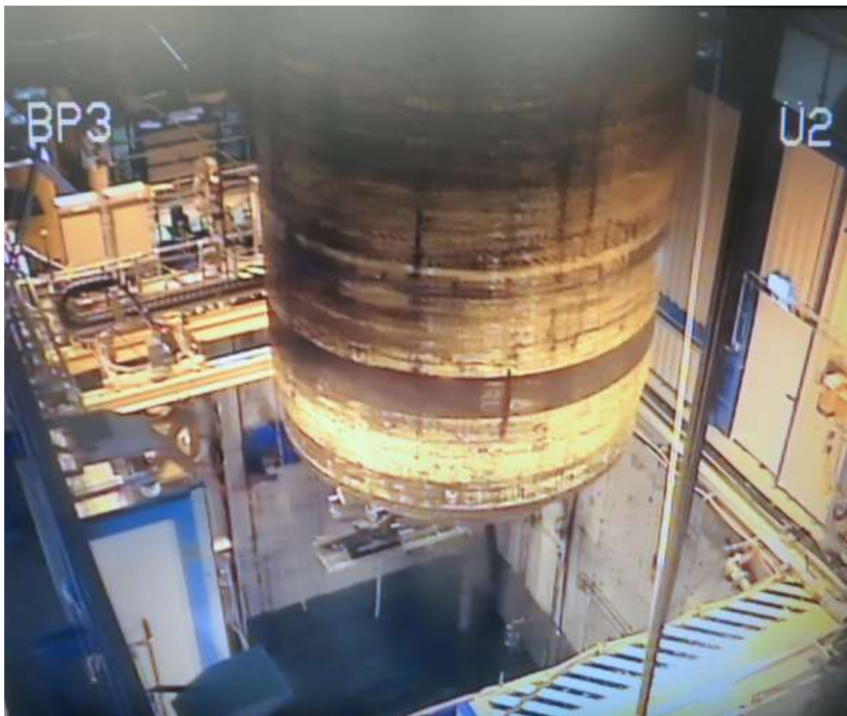
Fig. 4. RPV above the wet cutting area right before the settling
