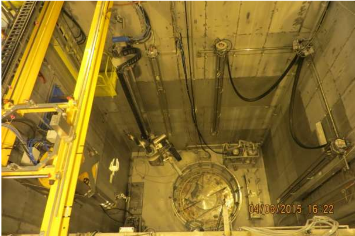
Fig. 2. Wet cutting area room 01.202 with dismantling equipment before lifting the RPV
