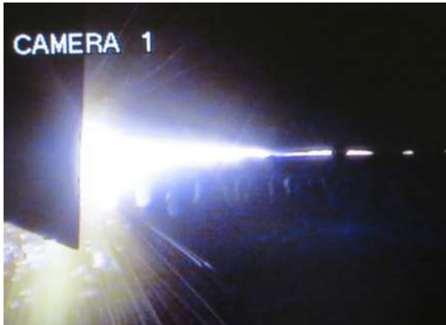
Fig. 5. Kerf at the RPV, heat protection metal sheet on the burner
