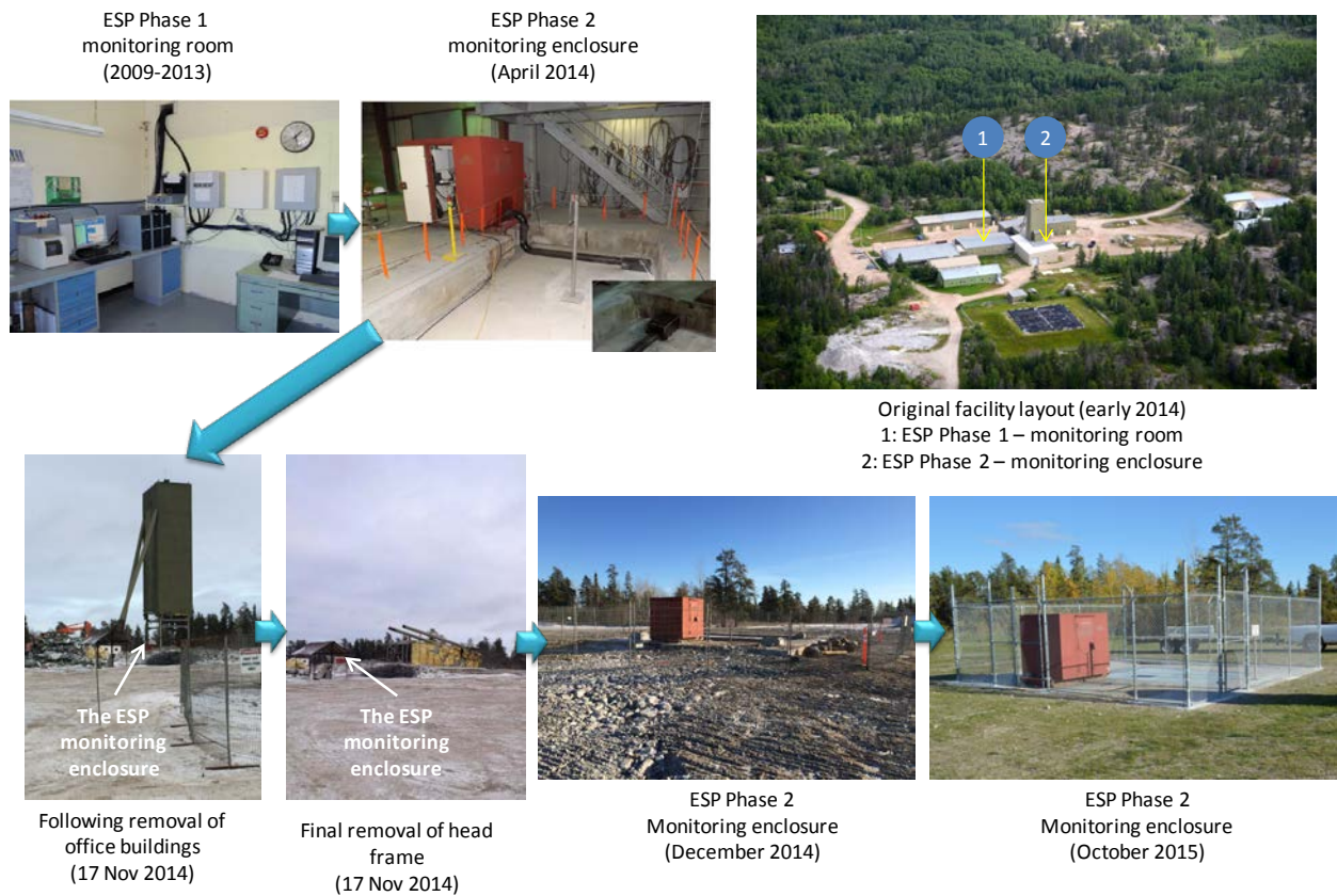
Fig. 2. ESP Monitoring Enclosure Near the URL Concrete Shaft Cap
