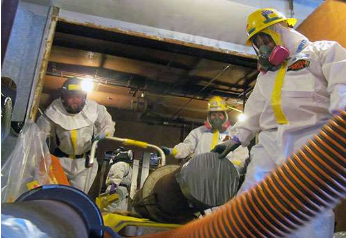
Fig. 4. Deactivating K-27 – Process Piping Removal.
