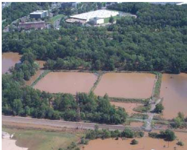
FIGURE 4. FLOODING OF IMPOUNDMENTS FROM HURRICANE IRENE AT AMERICAN CYANAMID SITE [6].
