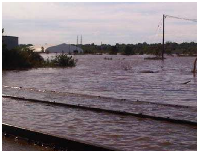
FIGURE 3. RARITAN RIVER FLOODING AMERICAN CYANAMID SITE NORTH AREA WITH FIVE FEET STANDING WATER [6].
