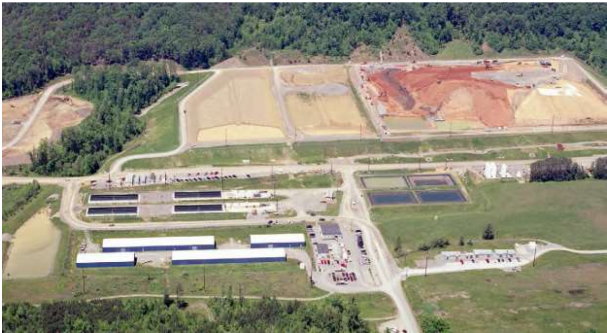
FIGURE 6. EMWMF LOCATED IN BEAR CREEK VALLEY, ORR, TN.
