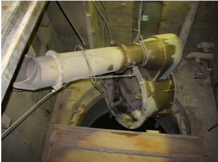
Fig.3. Removing of the low support of the MR reactor
