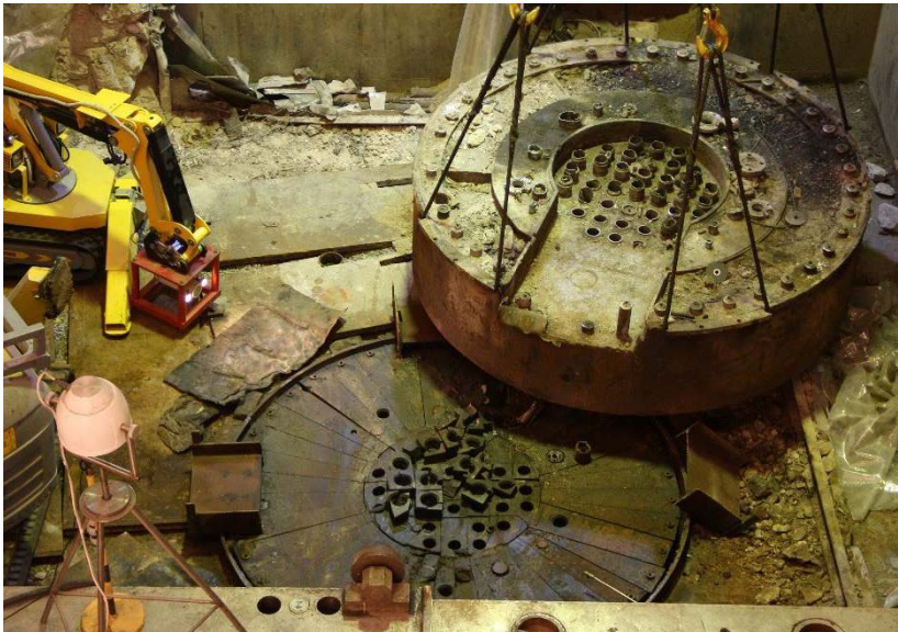
Fig.5. Graphite laying and top concrete covering of the RFT reactor.
