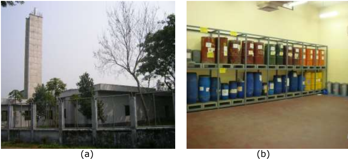
Fig. 3. (a) Central Radioactive Waste Processing and Storage Facility (CWPSF) and (b) Stored Drums with RWs in the Storage Area of CWPSF.
