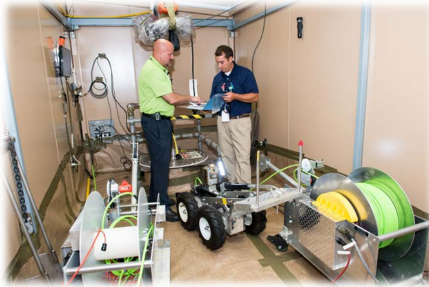
Fig. 12. Manway Room inside Permanent Hut
