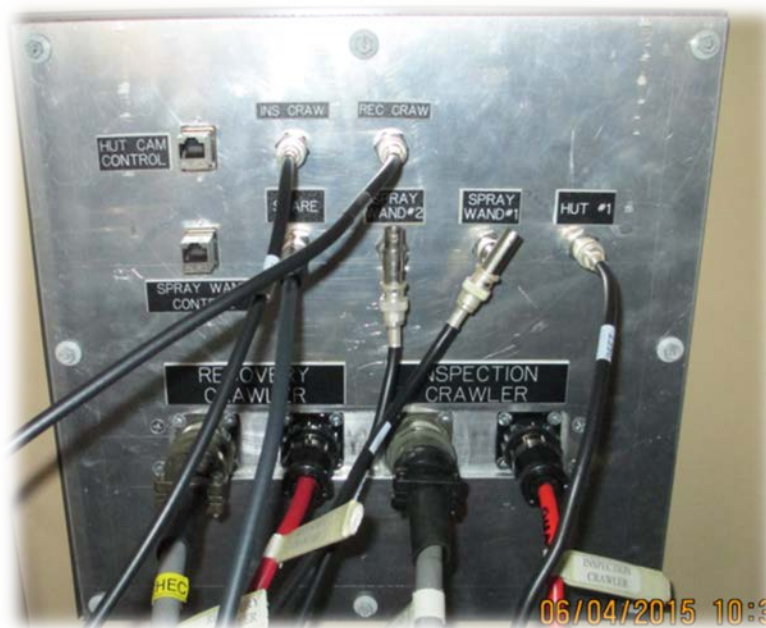
Fig. 13. Crawler Bulkhead inside Permanent Hut
