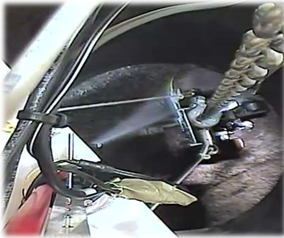
Fig. 21. Decontamination of the RC inside Exhaust Tunnel
