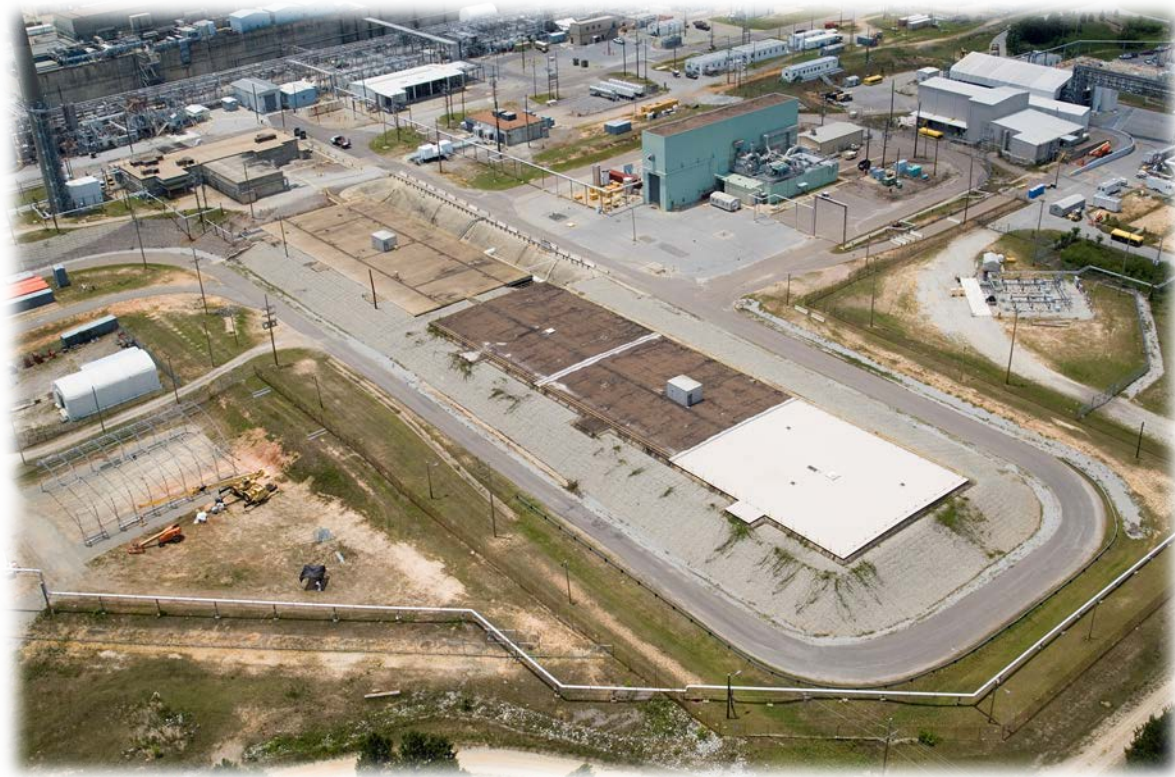
Fig. 2. H-Canyon Sand Filter Facility
