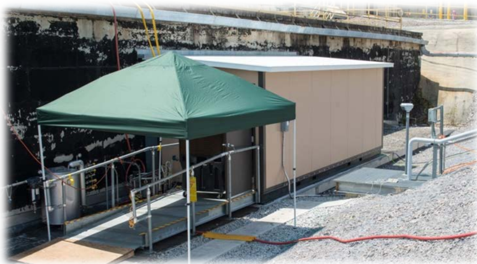
Fig. 8. – Permanent Hut for Crawler Work
