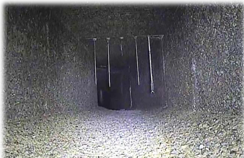
Fig. 18. Ramp up from Sand Filter inside Exhaust Tunnel
