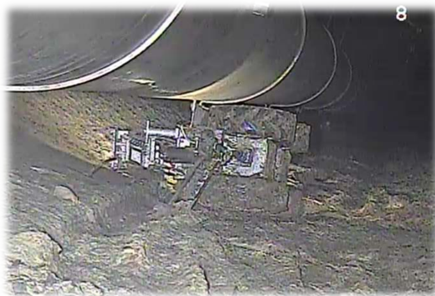
Fig. 20 c. Final Location of IC inside Exhaust Tunnel
