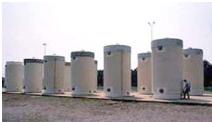
Fig. 4. View of large vertical DSCs containing HLW.
