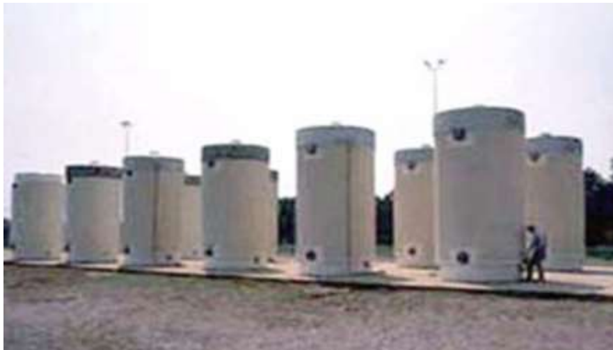
Fig. 6. One type of dry-storage containers (DSCs) for HLW in the USA.
