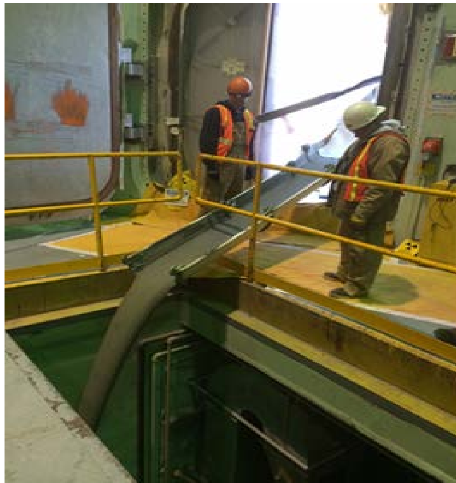
MFC-767 Grout pouring into basement area
