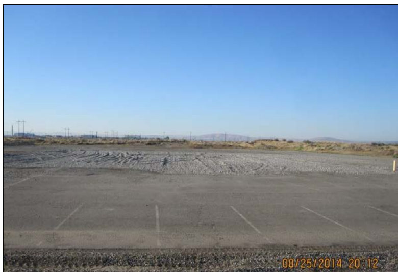
Site after Backfill, August 25, 2014
