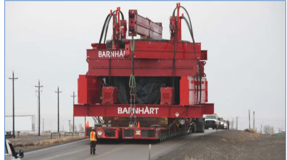
Reactor and bioshield monolith removed and transported to ERDF January 2014
