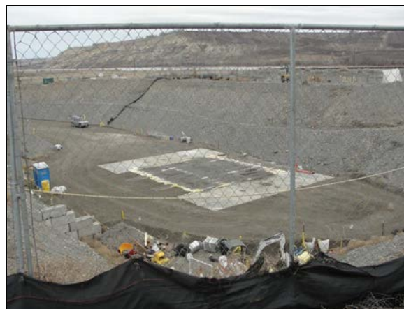
Vault Excavation February 18, 2014
