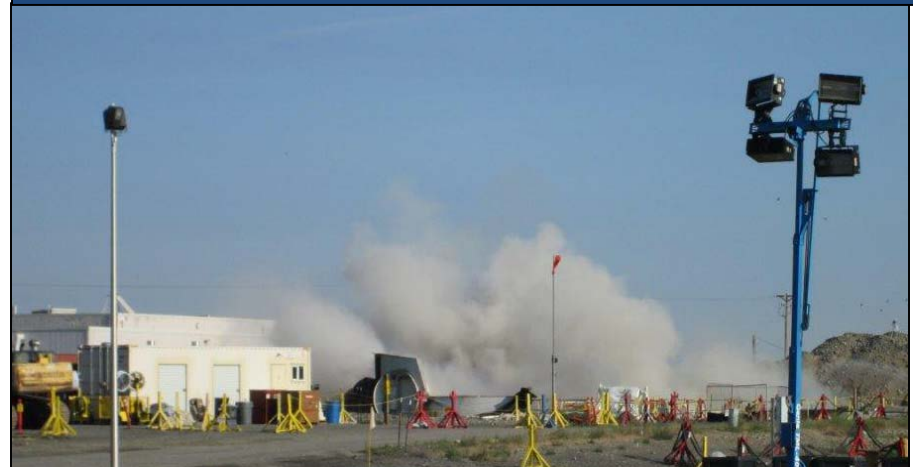
Explosive demolition of contaminated vessel August 2014
