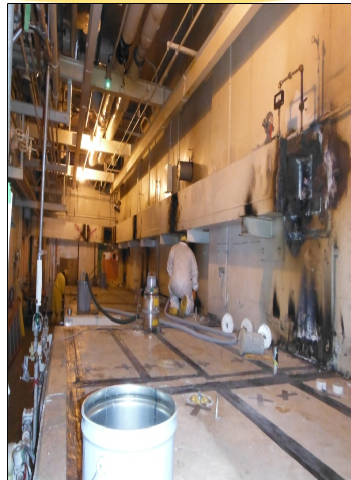
UWA Shielded Pipe Chase
