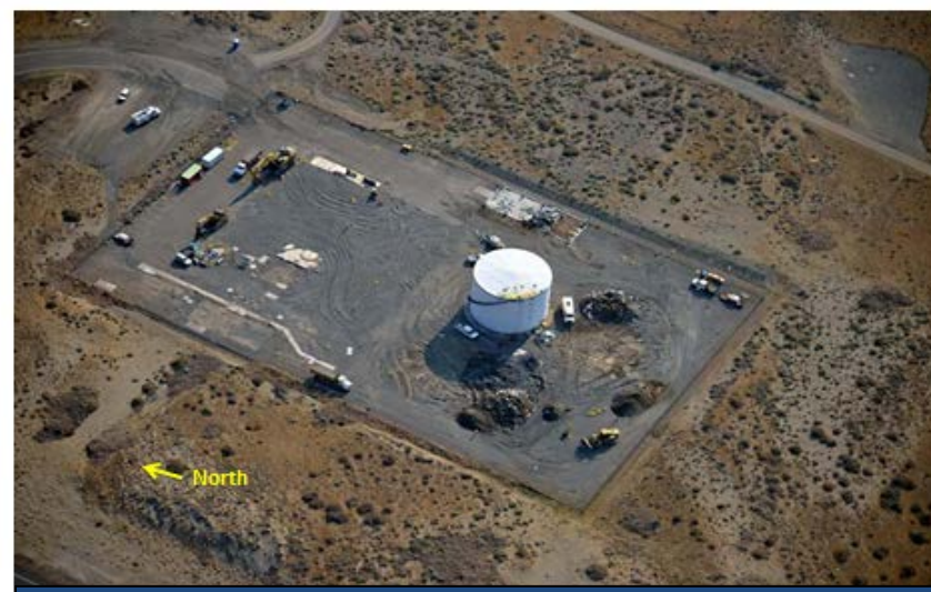
During Demolition, July 2014
