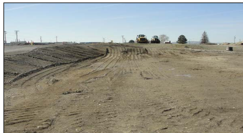
Site Completion April 30, 2014
