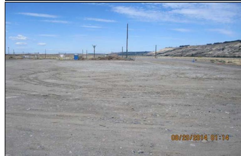
Complex after backfill August , 2014
