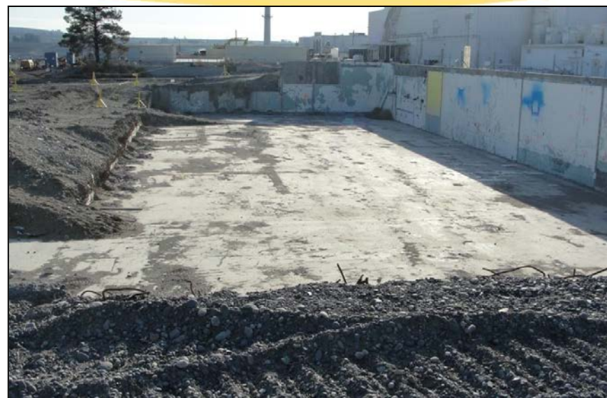
Basement prior to Backfill, May 2014
