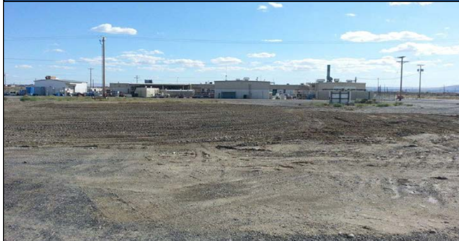
Site Completion following backfill, September 11, 2014
