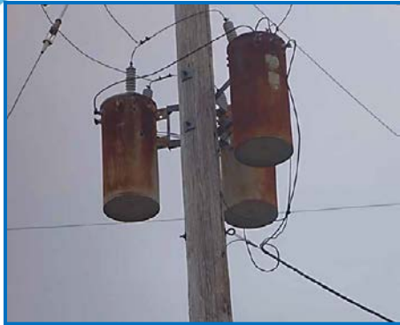
A-Area Pole Transformers
