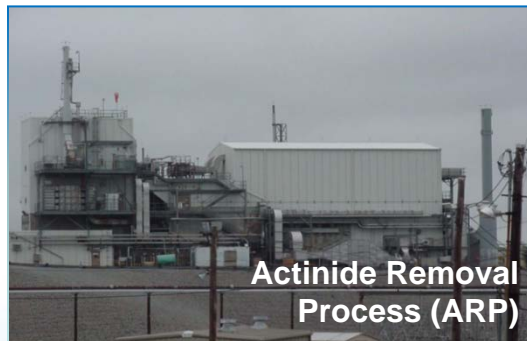
Modular Caustic Side Solvent Extraction Unit (MCU)
