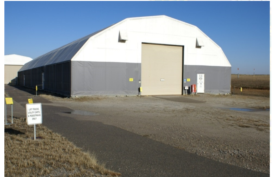
Typical TRU Waste Storage Pad (Pad 14)
