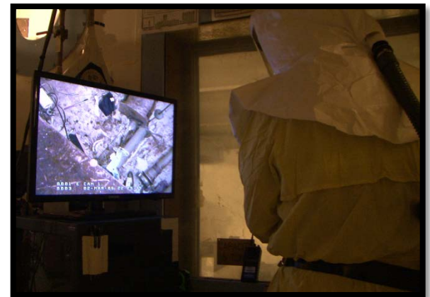
Crane operator moving pencil tanks for size reduction
