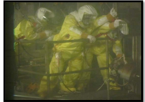
Employees repairing the crane in the PRF canyon
