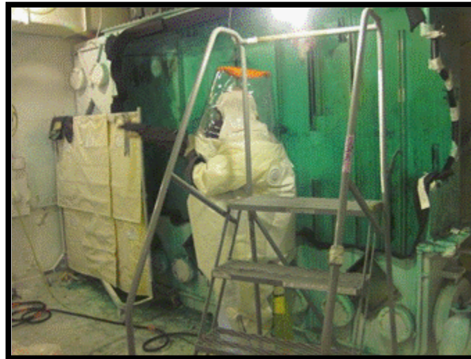
Employee size reducing WT-3 glove box in 242-Z
