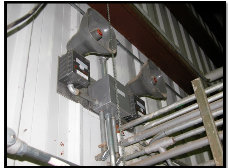
Criticality System Horn – As TSR controls are reduced, maintenance of these systems will be reduced and eventually discontinued
