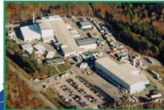
Bear Creek Operations, Oak Ridge, TN
