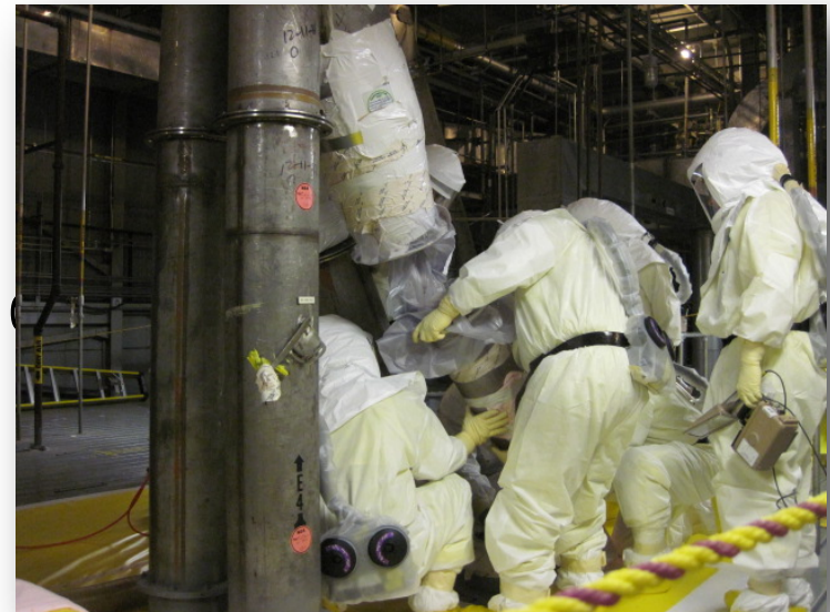
Crews removing ventilation ductwork, heavily contaminated after years of plutonium production
