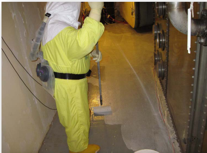
Applying fixatives to contaminated items
