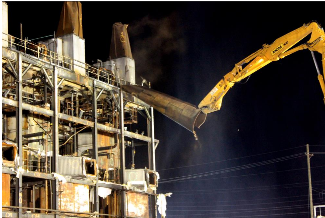
X-600 Steam Plant Demolition
