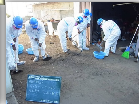
Garden: removal of topsoil
