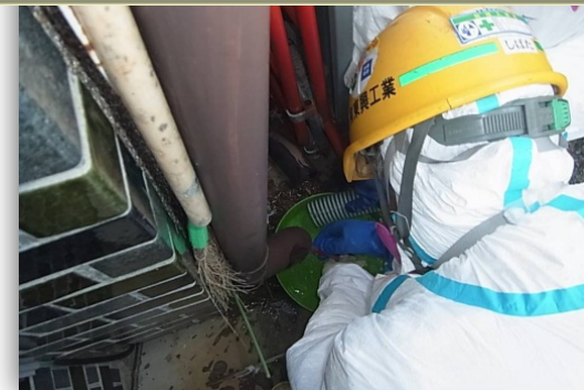
Gutter (vertical): high-pressure water cleaning
