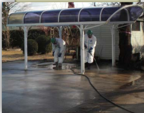
Concrete floor: High-pressure water cleaning
