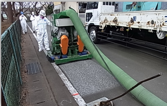
Surface grinding by shot blast
