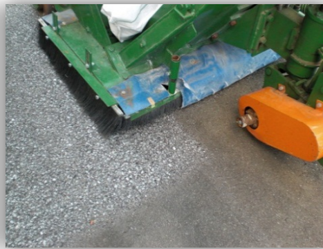
Surface grinding by shot blast
