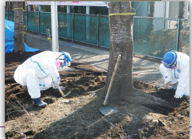
Removal of topsoil
