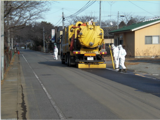
High-pressure water cleaning by vehicle for recovering functions of water drainage pavement
