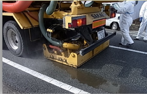
High-pressure water cleaning by vehicle for recovering functions of water drainage pavement
