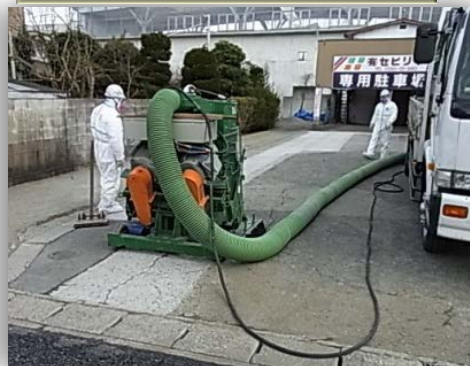
Concrete floor: Shot blast
