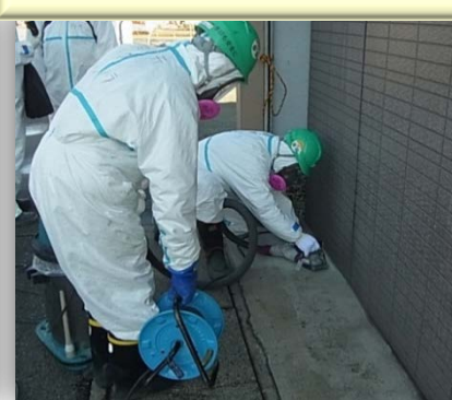
Concrete floor: Surface grinding machine
