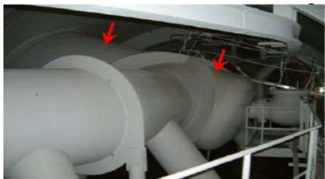
Access location in vent tube for Inflatable Bag Tool and Grout Tool
