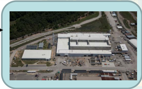
SWPF (under construction)
