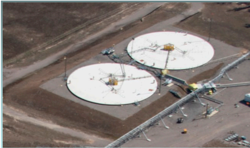
SDU 2: Placed into Service in 2011; Filled in 2013
