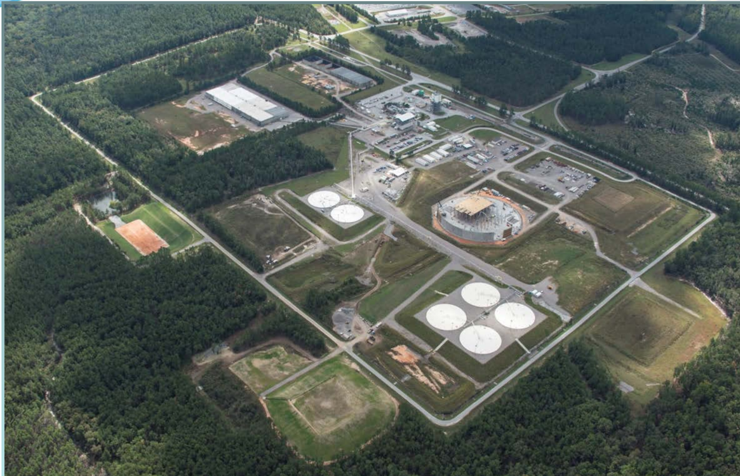
Savannah River Site
