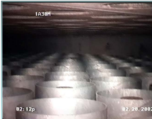
Inside vault looking across rows of canister supports
