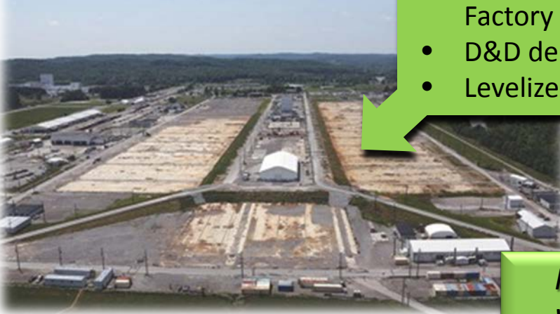
K-25 demolition completed
