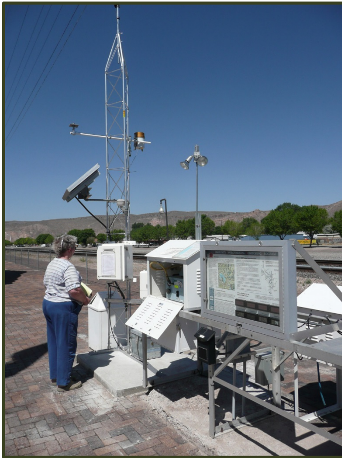
Station in Caliente, NV
