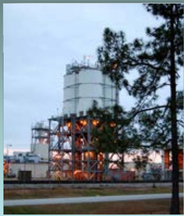
Grout Waste Form Development
