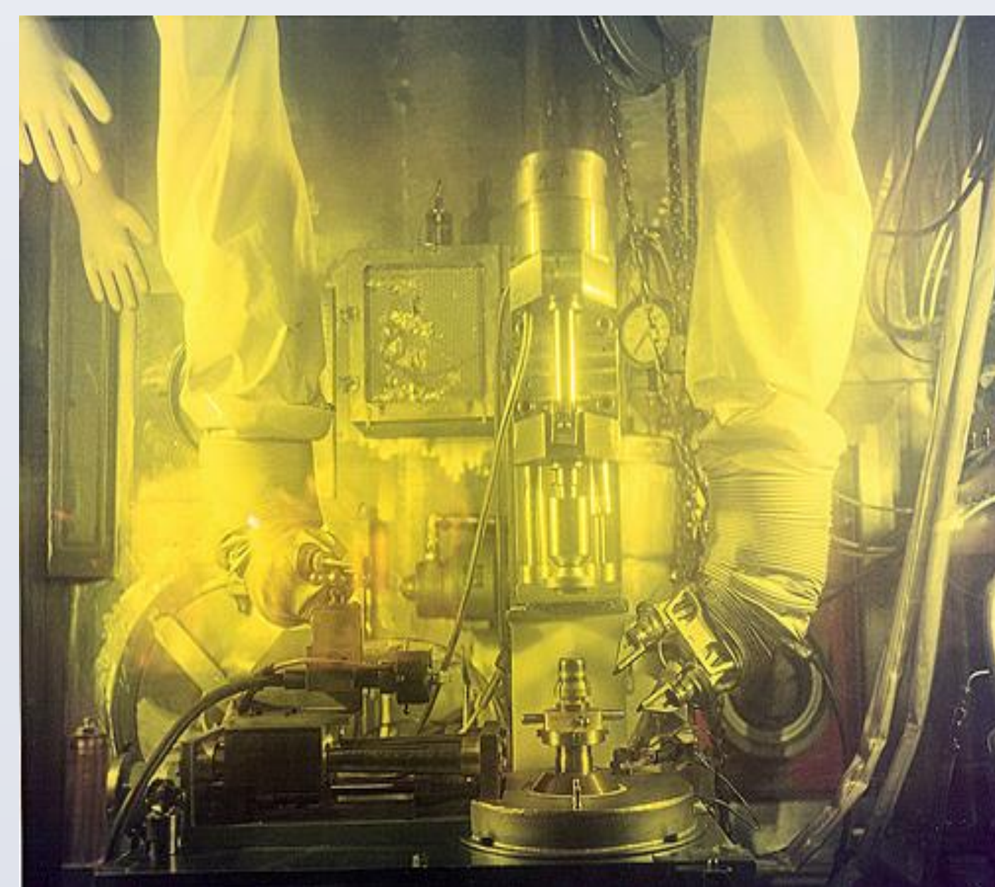
Figure 1. Interior of glove box in Building 235F at Savannah River Site
