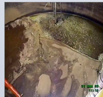
Figure 4. SRS Tank 19 Before Cleaning
