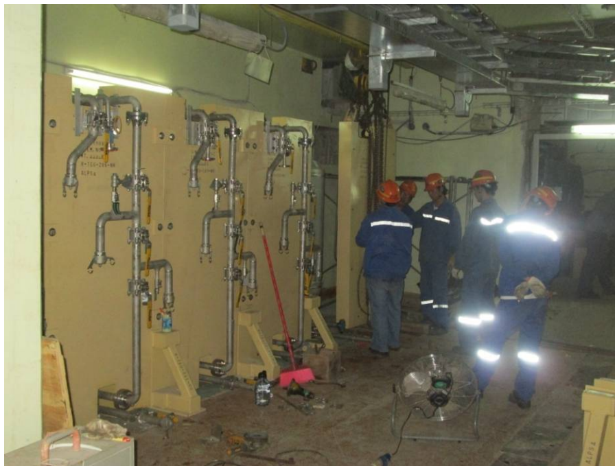
Fig. 4. ES ALPS system during installation
