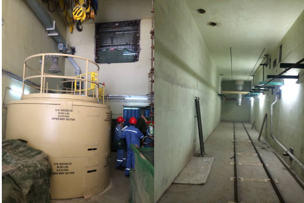
Fig. 5. TES during installation
