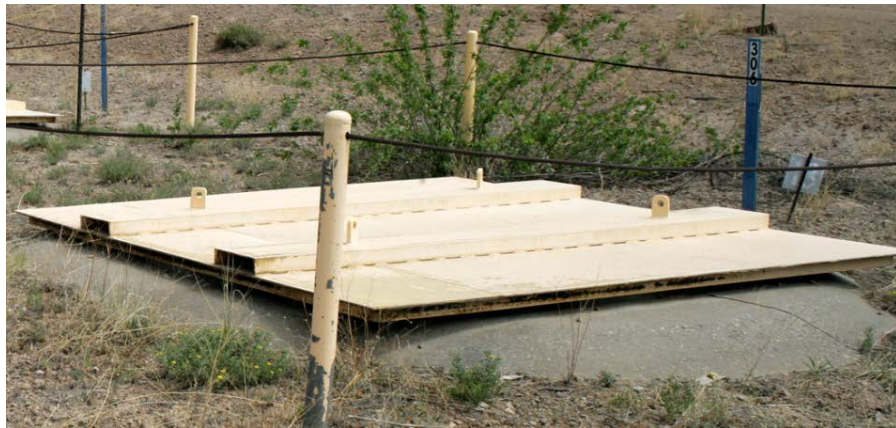
Fig. 10 Shaft Cover and Domed Concrete Collar at Top of Shaft.
