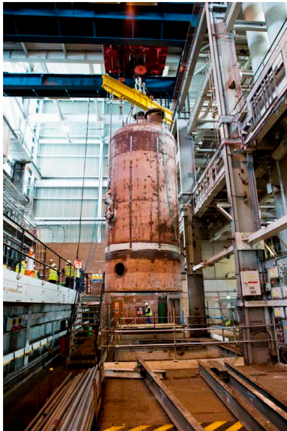
Figure 9: DDT Lifted from Pit
