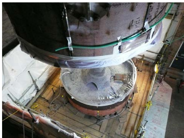
Figure 11: Residual Sodium in the Bottom of a DDT is Exposed after Cutting and Lifting Away the Tank Top
