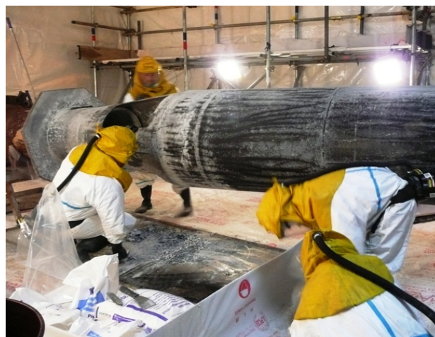
Figure 16: Removing Sodium from Centre Dump Tube
