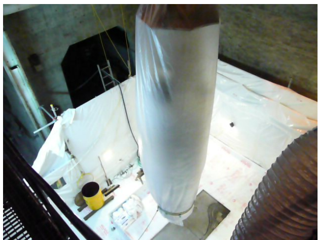
Figure 15: Lowering Centre Dump Tube into Processing Area
