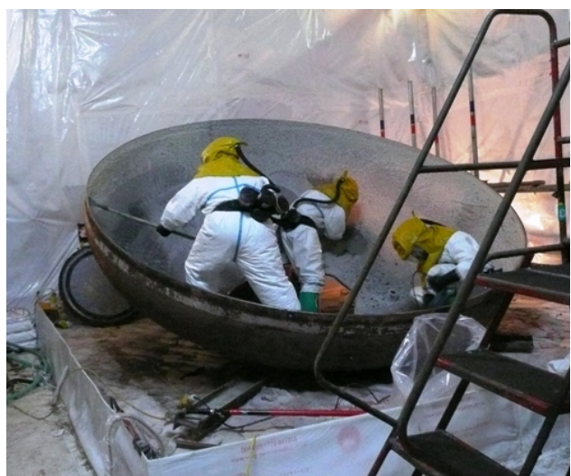
Figure 13: Scraping and Wiping a Top Dome
