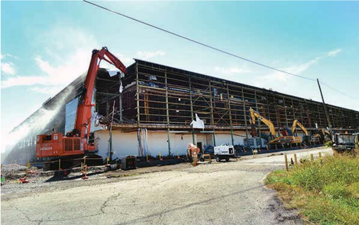
Figure 3. Beginning demolition of the 17-acre K-31 plant.
