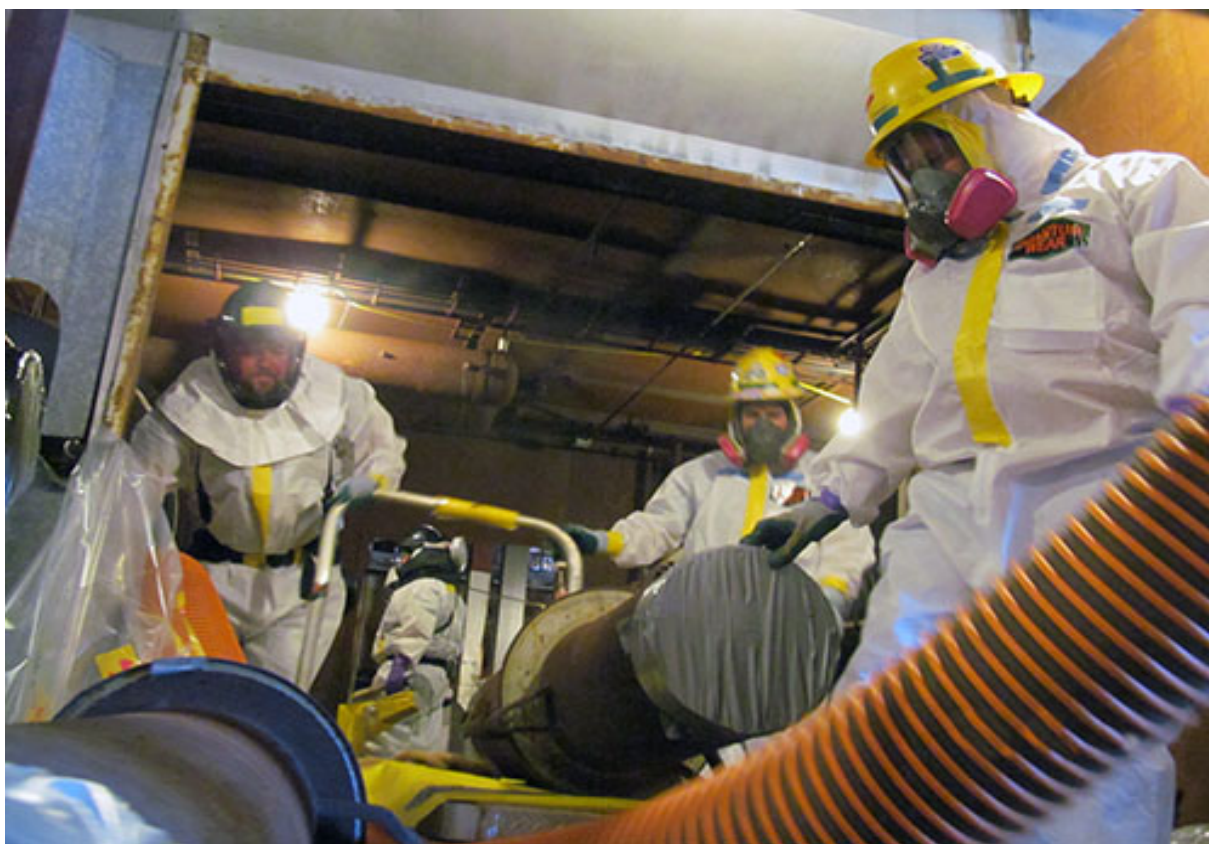
Figure 4. Deactivating K-27 – Removing Process Piping
