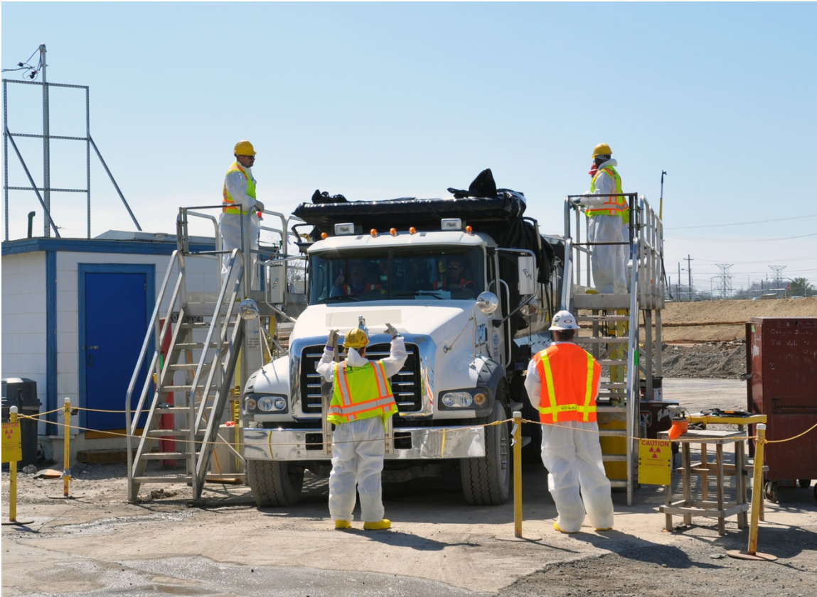
Figure 2. Removal of remaining demolition debris from the K-25 footprint.
