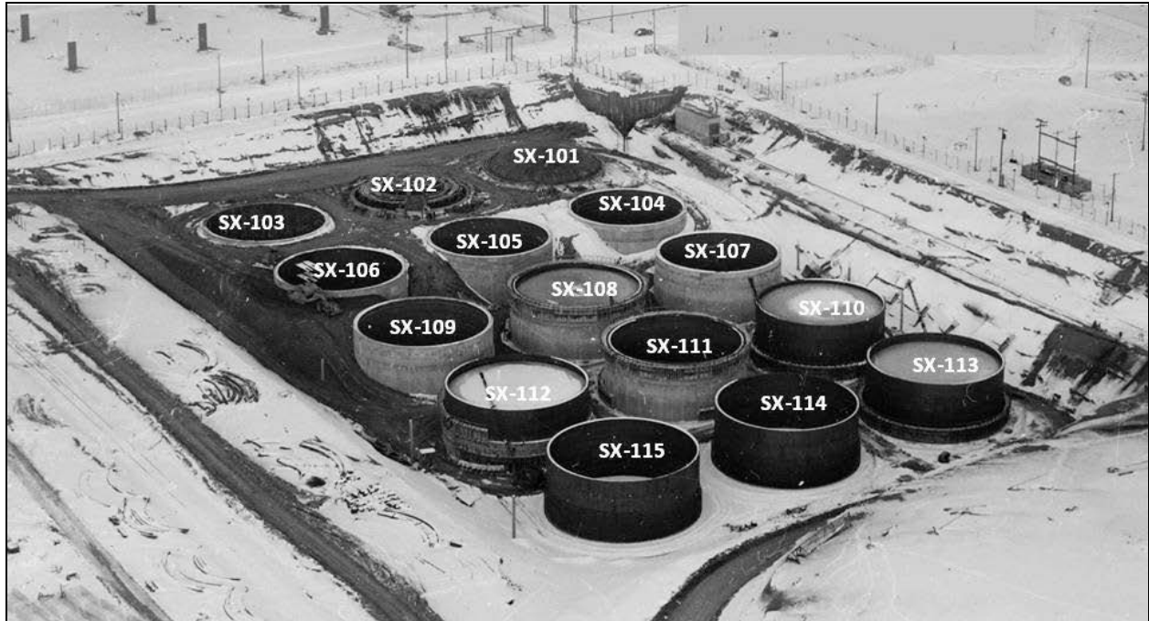
Fig. 3. SX Farm Construction Photograph Taken January 20, 1954
