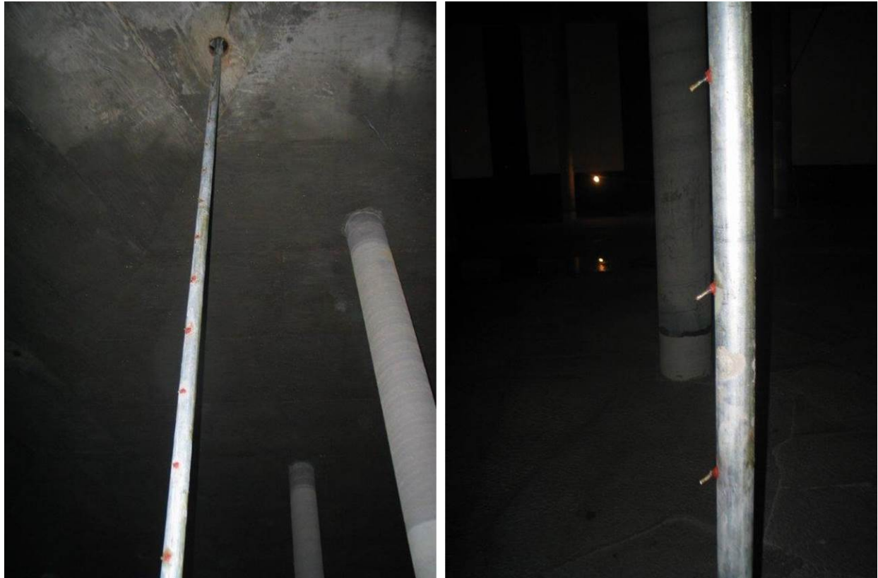
Figure 2: Vertical thermowell array in SDU.
