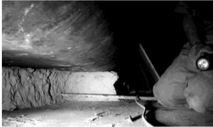
Figure 3: Refractory Repair Operations in 241-AY Tank Farm
