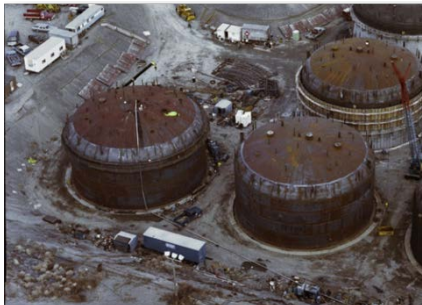
Primary Tank Hydrostatic Test
