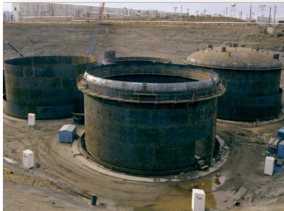
Primary Tank Walls
