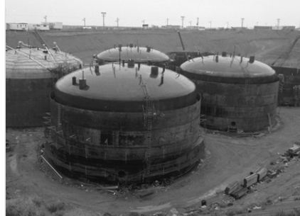
Sec. Liner Walls & Prim. Tank Dome
