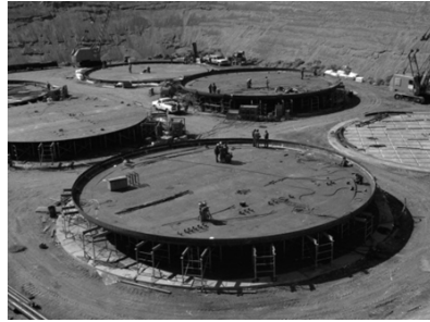
Secondary Liner Bottom
