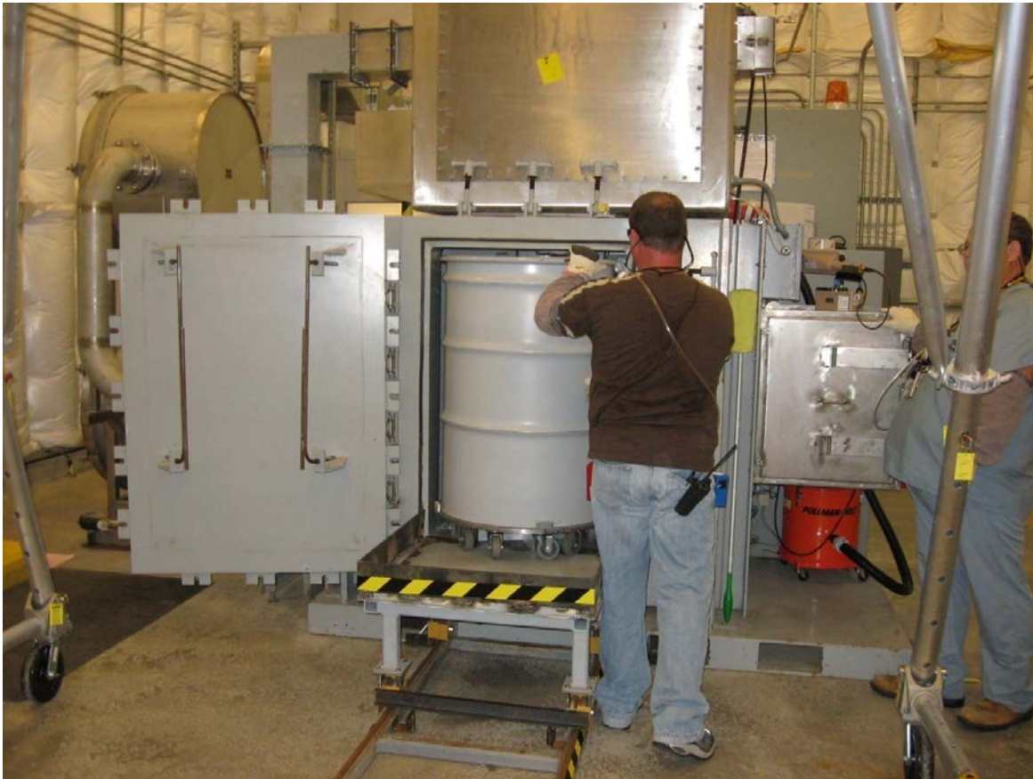
Fig. 2. Operator Inserting Overpacked Drum into DVS Cabinet
