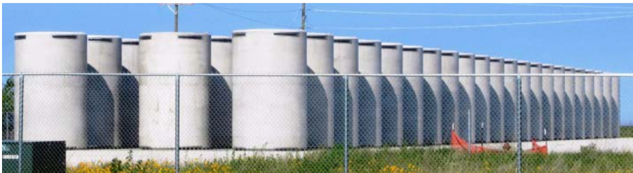
Figure 1 – Vertical Storage Overpacks
