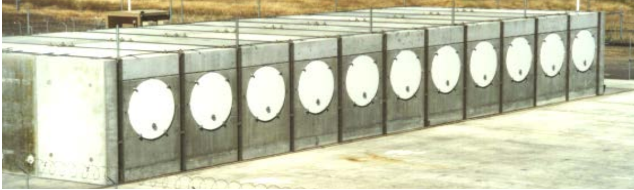
Figure 2 – Horizontal Storage Modules
