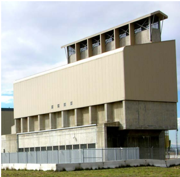
Figure 5 – Fort St. Vrain ISFSI Vault Storage
