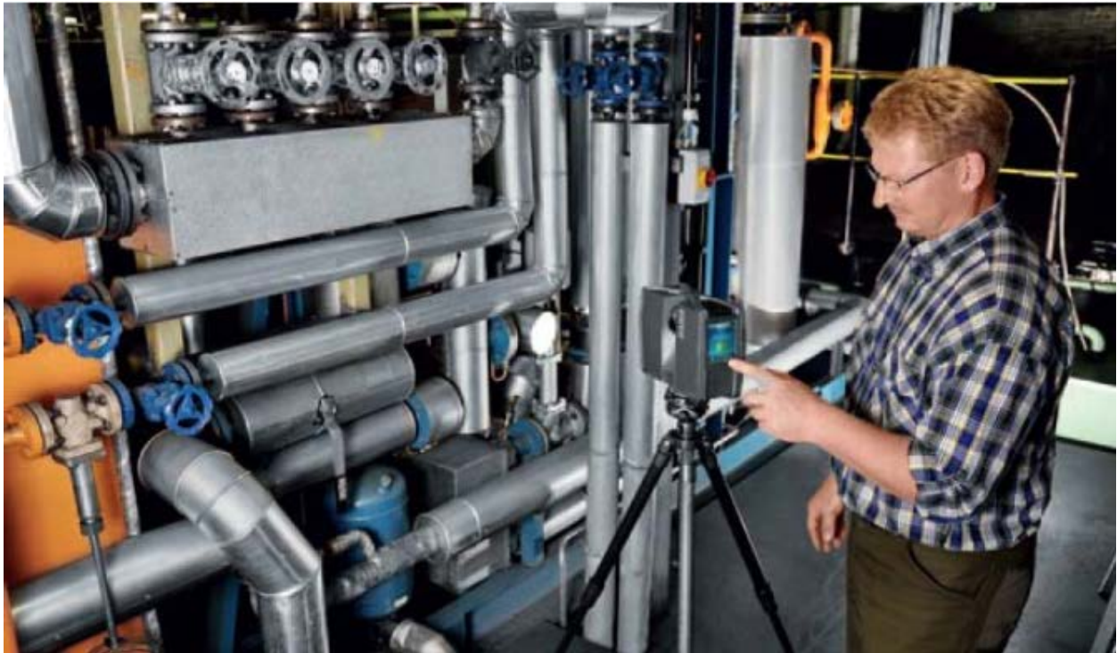
Figure 1 – Point Cloud Scanner
