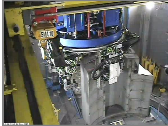
Fig. 6 Cutting of a primary shielding block by using the band saw
