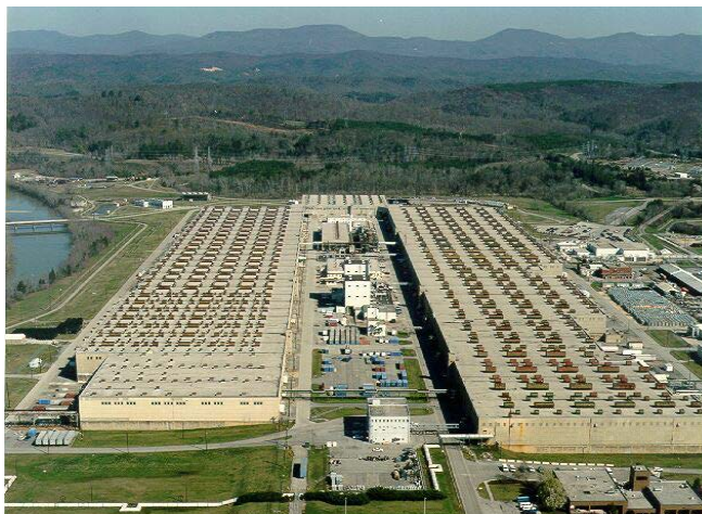
Fig. 1. K-25 Prior to Demolition
