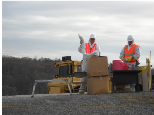
Fig. 9. Workers Prepare to Place Sorbent "Pigs" in Truck Bed
