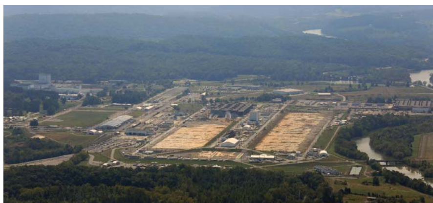
Fig. 2. K-25 During Start of Final Demolition (September 2013)
