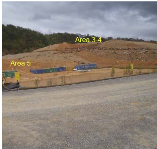
Fig. 6. View of "High and Dry" Placement Area
