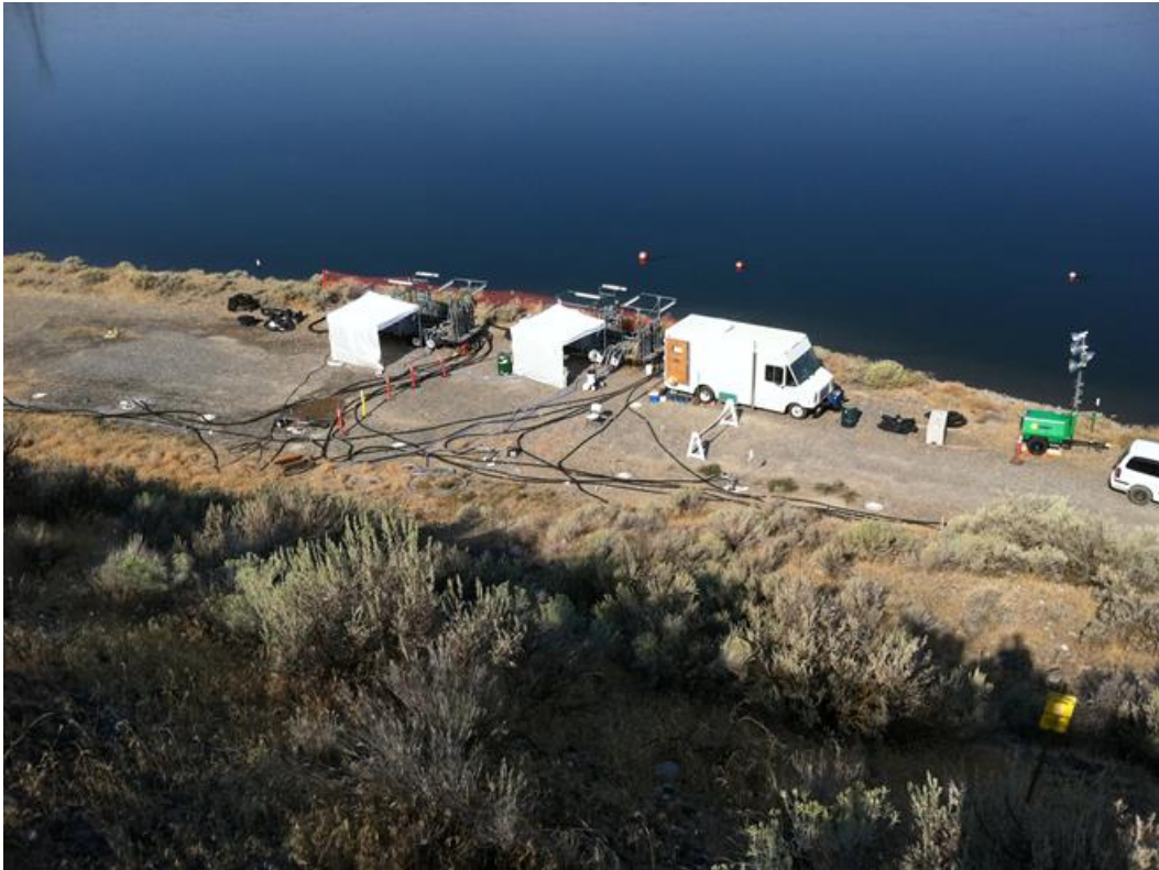
Fig. 6. Apatite Chemical Injection Skid Setup.
