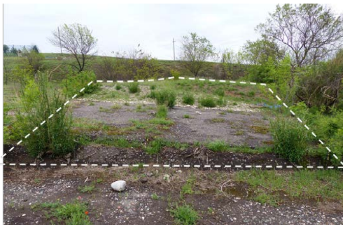
Figure 1: Surface area of the two vaults, in the foreground the surface of the asphalt layer can be seen and in the background the partly soil covered end of the vaults (width ca. 10 m, length 22 m).
