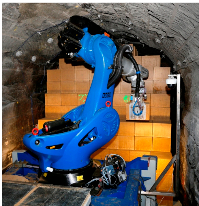
Fig. 9. Backfill installation robot operating in the Äspö HRL.
