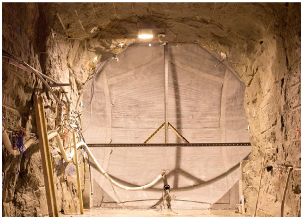
Fig. 10. The constructed deposition tunnel end plug at Äspö HRL.
