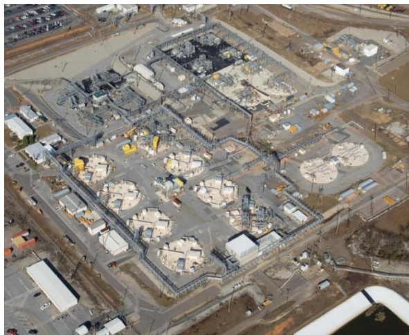
Fig. 2. SRS F-Tank Farm
