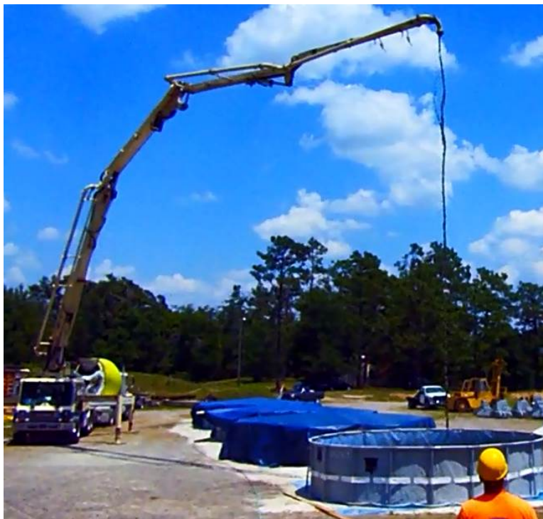
Figure 5 – Grout Drop Testing (Forty-Two Foot Free Fall)
