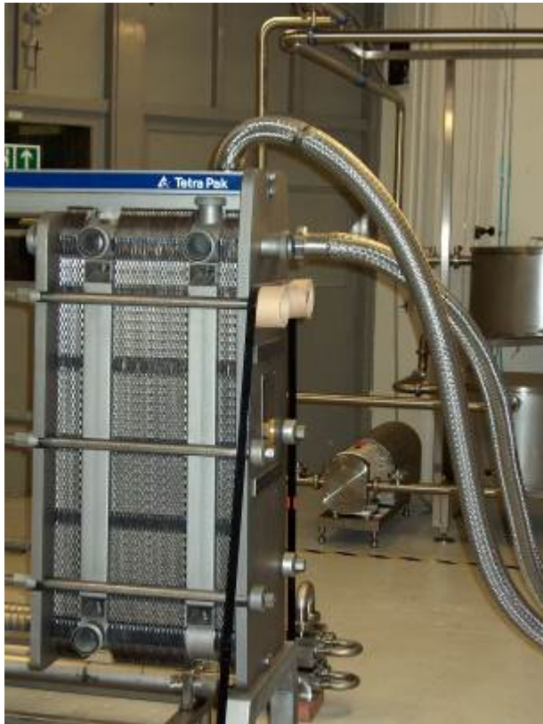
Figure 5. Ice pigging in a small industrial plate heat exchanger.
