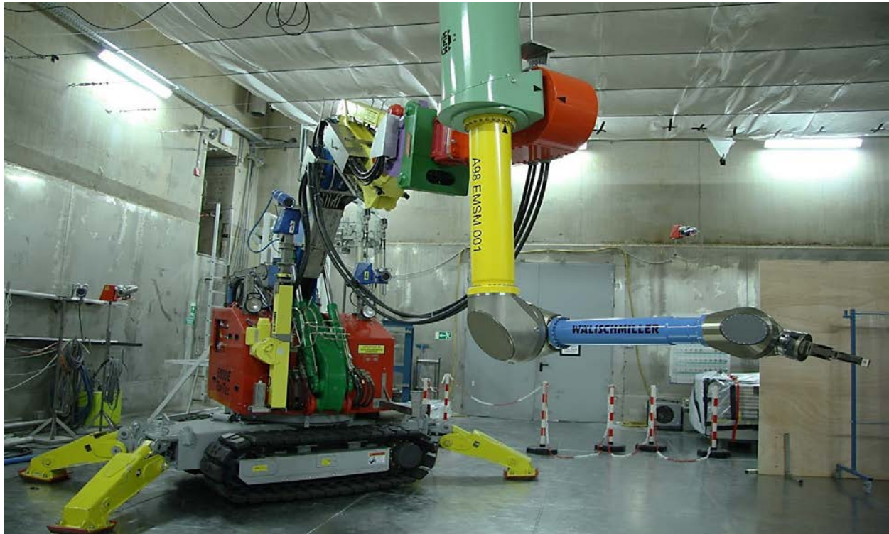
Fig. 4. Photograph of the robotic system TELBOT ® and the excavator
