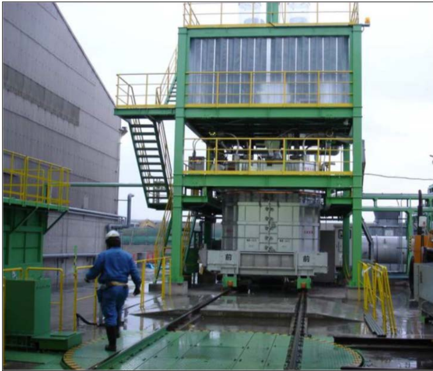
Fig. 1 Ten tonne ICV Melter during waste treatment operations.
