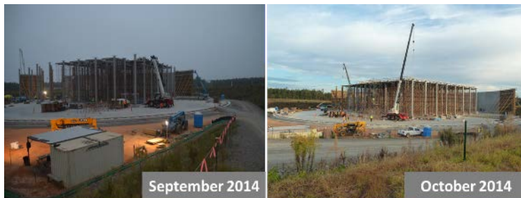
Fig. 4. SDU 6 Under Construction
