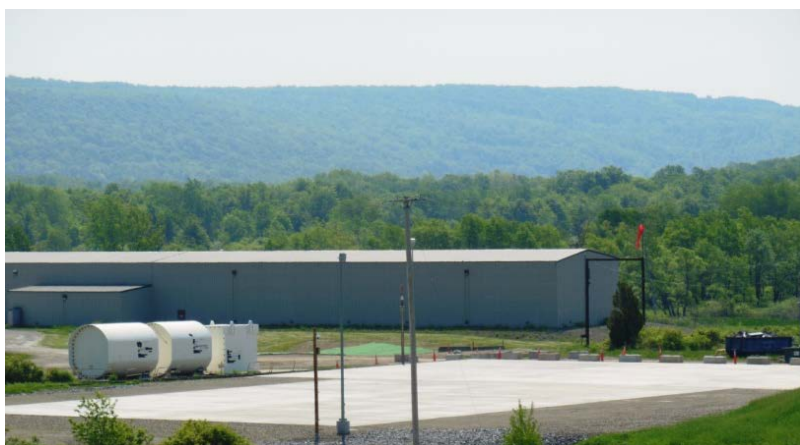
Fig. 5. The completed storage pad and approach apron.
