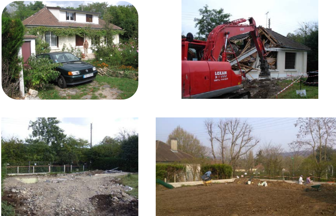
Figure 3: remediation of the polluted site in Gif sur Yvette
